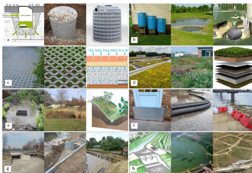
Figure 2. Examples of the water management systems shown in the survey: (a) soakaways; (b) rain harvesting systems; (c) permeable pavements; (d) green roofs; (e) bioretention systems; (f) temporary barriers; (g) diversion channels; (h) expansion basins.
