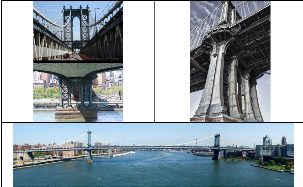
Figure 4.100 First photos during construction, opening and current conditions of the Manhattan Bridge.
