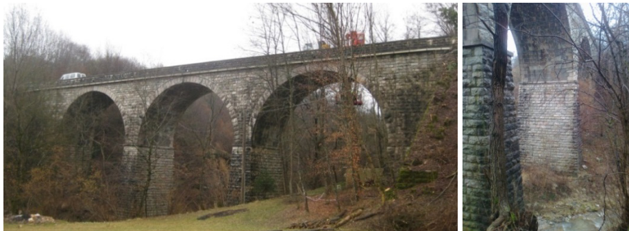
Figure 4.34 Panoramic view and piers of the Gresal Bridge.
