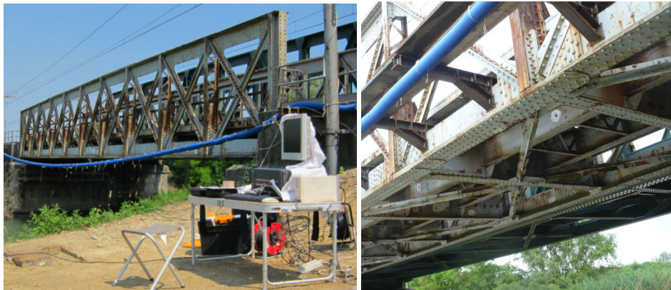
Figure 4.48 Views of the bridge during measurement operations and from below.
