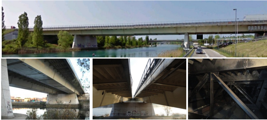
Figure 4.65 Views of the Mincio steel box girder bridge.
