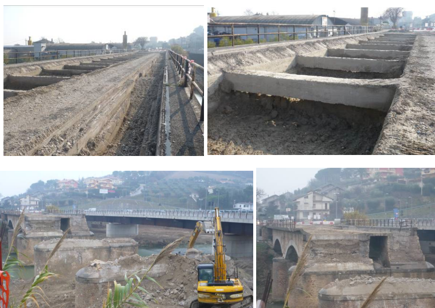
Figure 4.14 Sequential demolition process of the Tronto bridge.
