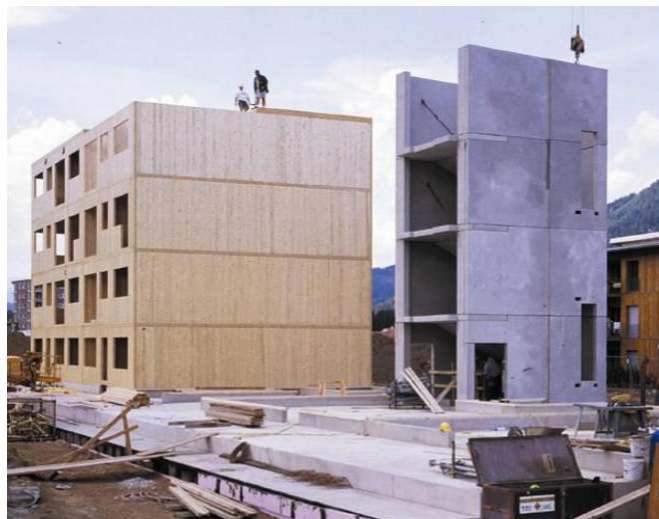
Fig. I.32 – Hybrid CLT-concrete system [I.20]
