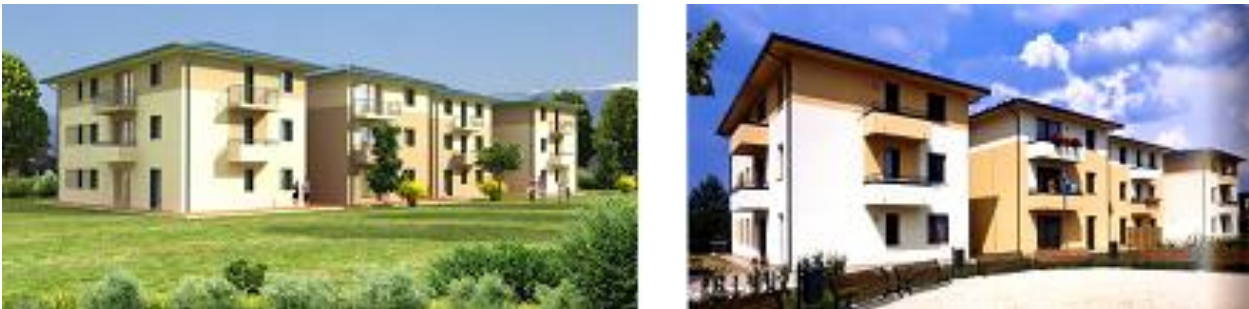
Fig. 5.7 – Views of the considered three storeys building.
