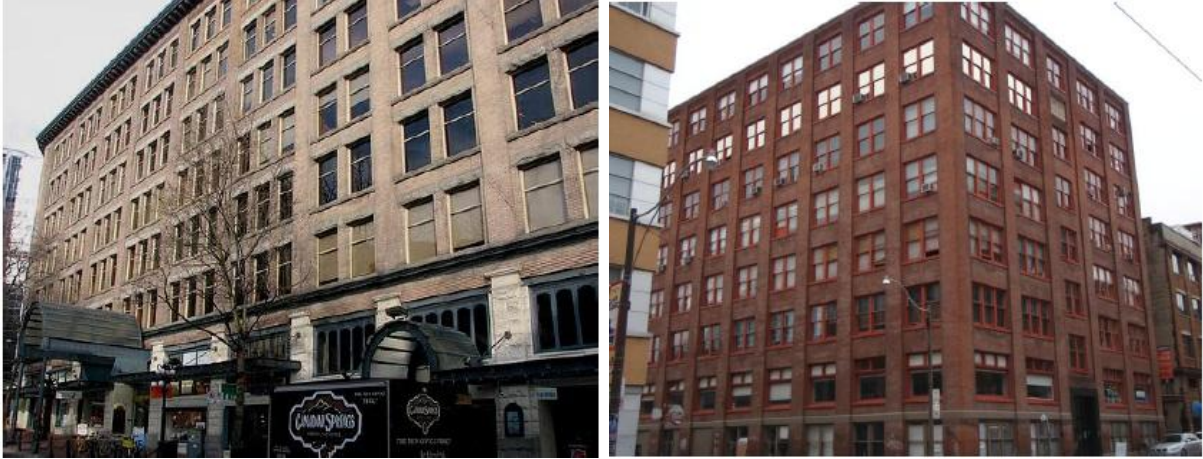
Fig. 1.18 – 8-storey brick-and-beam office buildings built in Vancouver in 1905 (left) and in Toronto in 1920 (right) [1.20]
