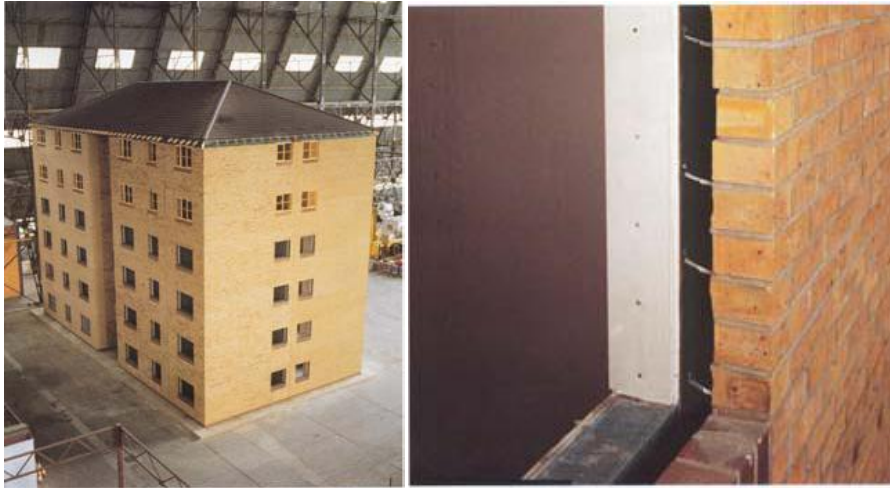
Fig. 7.2 – Brick Clad Timber Frame at BRE Cardington (left) and Typical Movement Joint (right) [7.1]
