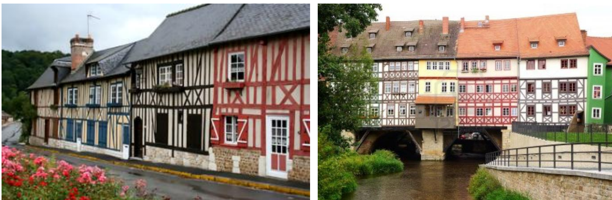
Fig. I.11 – Example of a “Colombage” building in France [I.15] (left) and of a “Fackwerk” building in Germany (right) [I.16]
