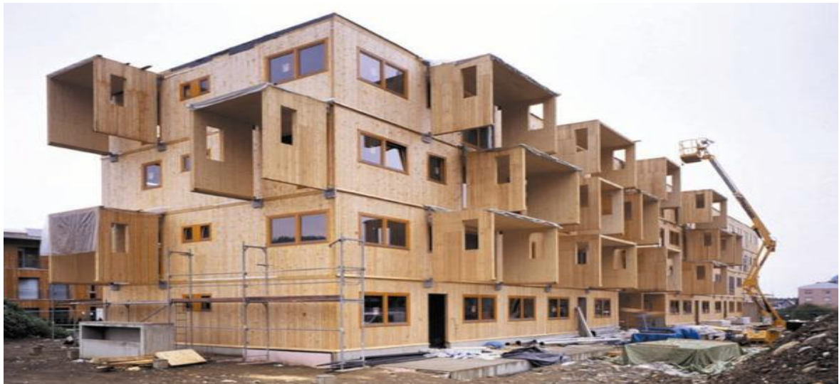
Fig. I.27 – Multi-family buildings in Austria [I.20]
