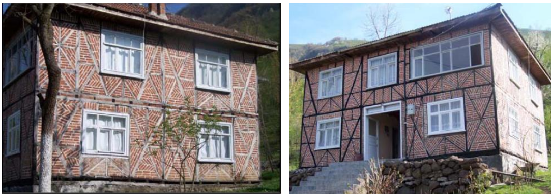
Fig. I.14 – Example of Brick infill himis structures [I.14].
