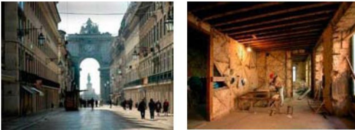
Fig. I.10 – Lisbon area rebuild with “Pompalino” system after 1755 (left) and typical “gaiola” wall [I.2]
