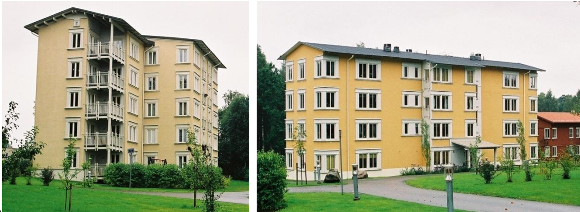
Fig. I.24 – Medium rise Platform Frame building in Växjö - Sweden [I.25]
