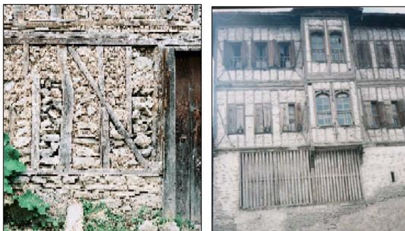
Fig. 1.13 – Example of stone infill himis structures [1.14].
