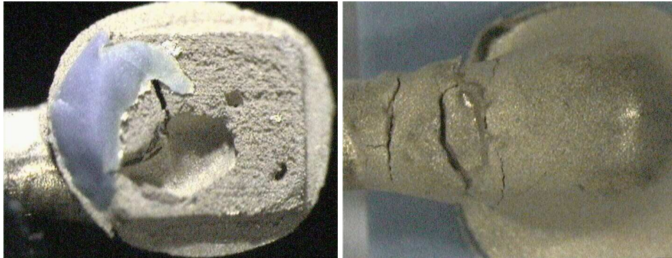
Figure 88 : the welded connection appears to be porous and cracked
