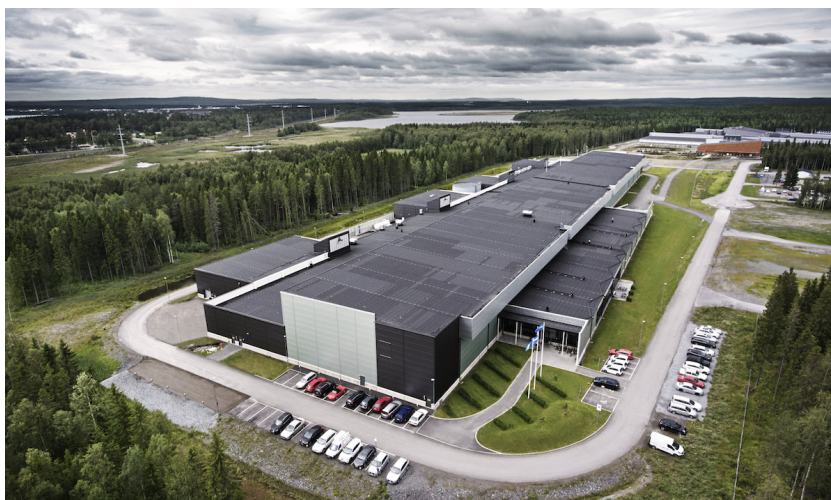
Figure 1.19: Aerial view of the 300 meters wide by 100 meters long Facebook Data Center in Luleå, Sweden.
