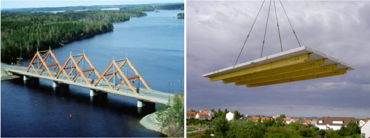
Fig. 1.1 – TCC bridge deck in Finland on the right [1.5] and TCC prefabricated floor on the left [1.6].
