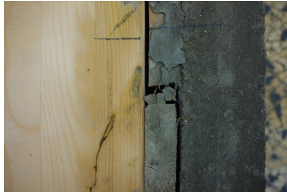
Fig. 2.23 – Localized failure of a specimen with interlayer (ID:LB_FT_5) observed at large displacements.
