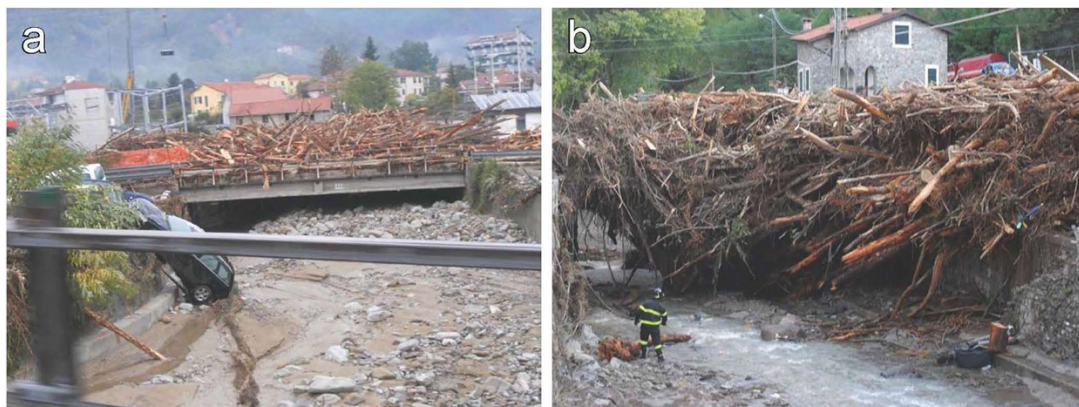
Figure 5: LW clogging in the Magra river catchment (Italy) after the 2011 flash flood (after Lucia et al., 2015).
