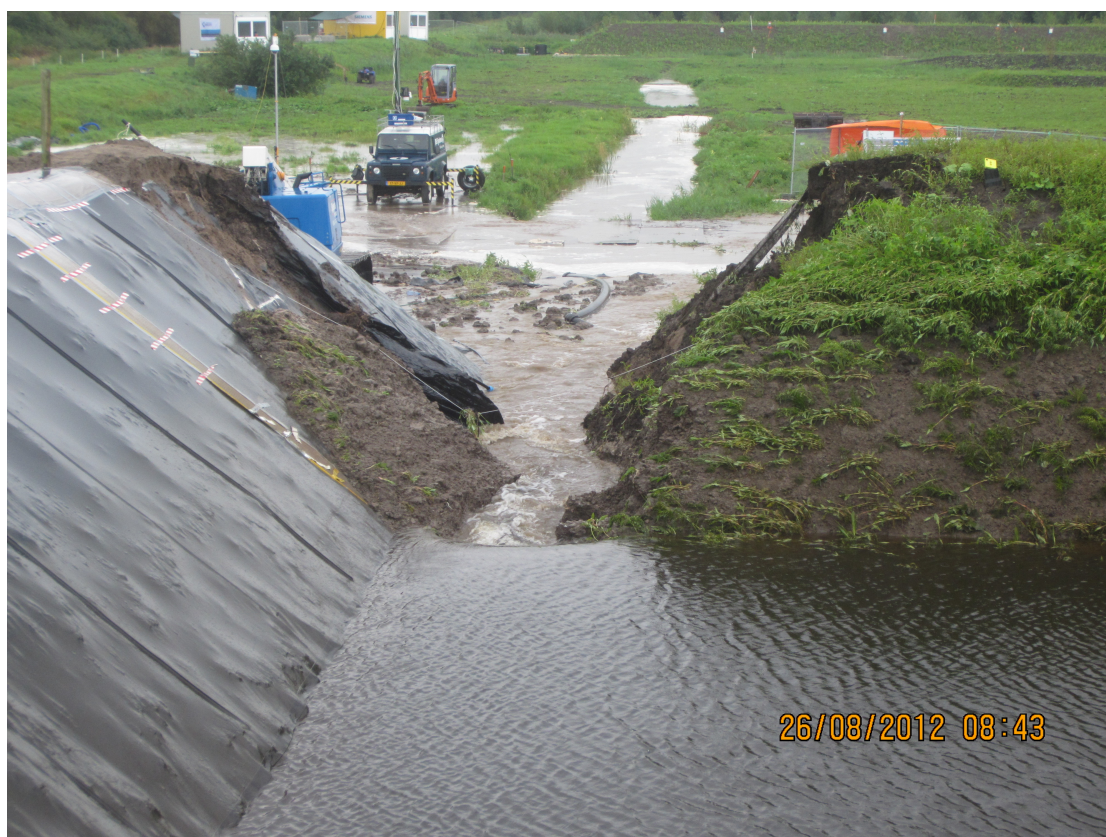
FIGURE A.30: Emptying of the upstream basin nearly complete
