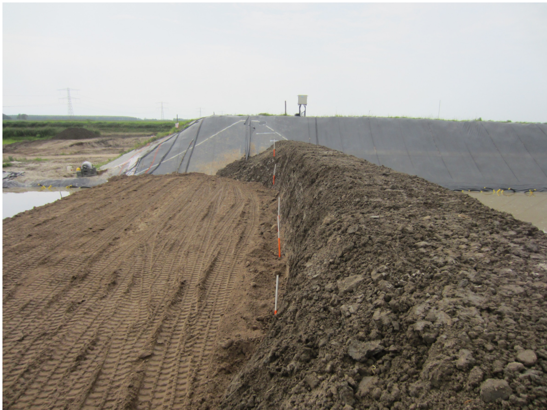
FIGURE A.17: Extra lump of clay placed near the sides in order to avoid failure at the ends
