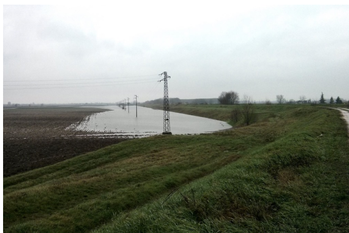
FIGURE 1.2: Heavy underseepage occurring at Vescovana, along the Gorzone river, in February 2014
