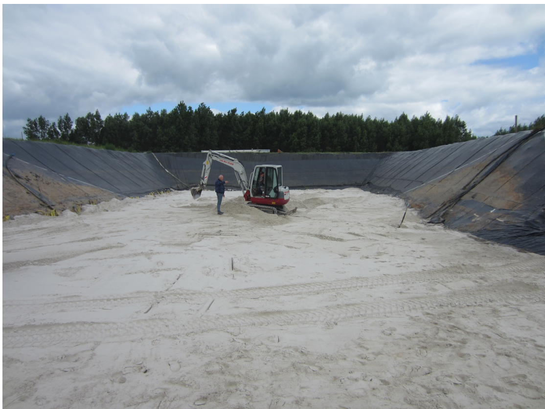
FIGURE A.6: Piping facility during deposition of the new sand
