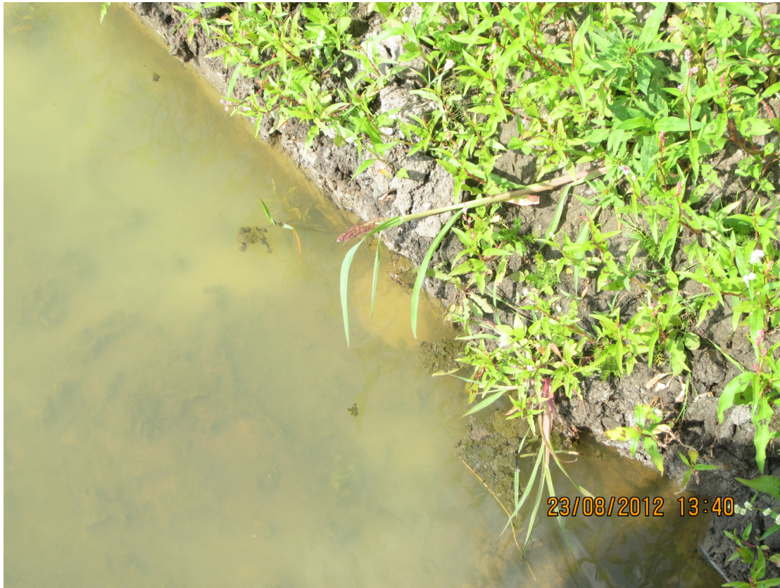
FIGURE A.21: First sand boil observed.
