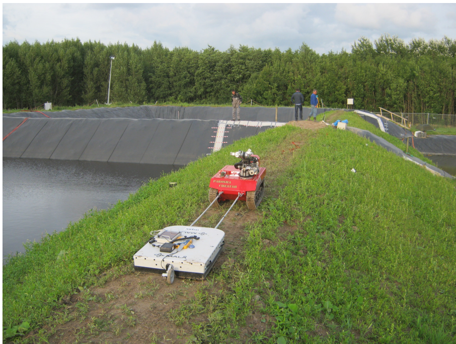
FIGURE A.20: Ground Penetrating Radar guided from a distance along the dike crest.
