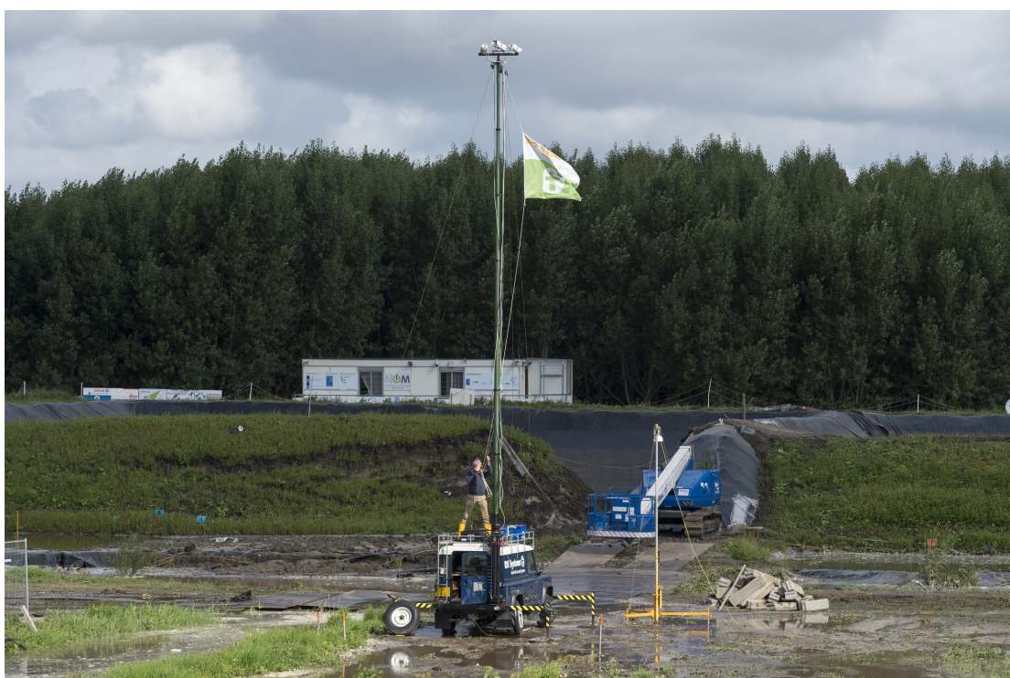
FIGURE A.12: Infrared cameras pointing to the downstream West and East slopes.
