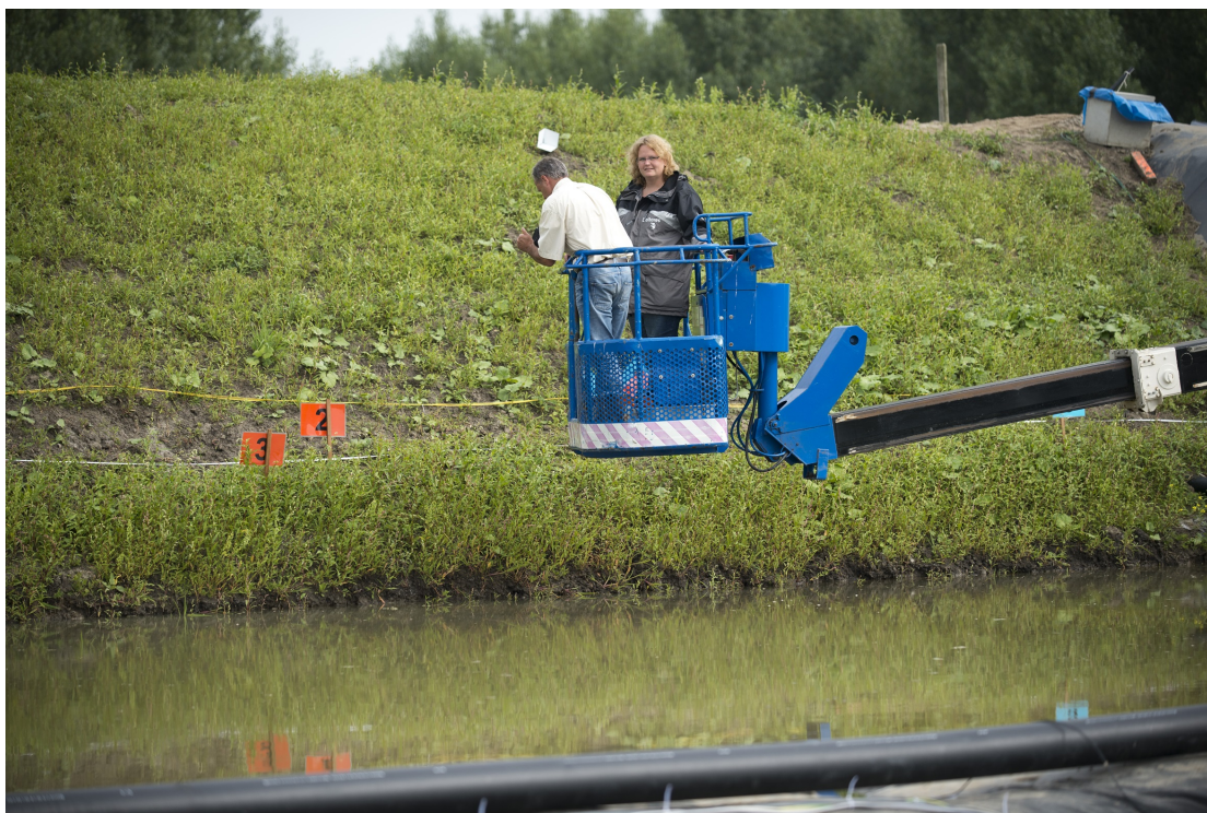
FIGURE A.11: Visual inspection performed from a crane.
