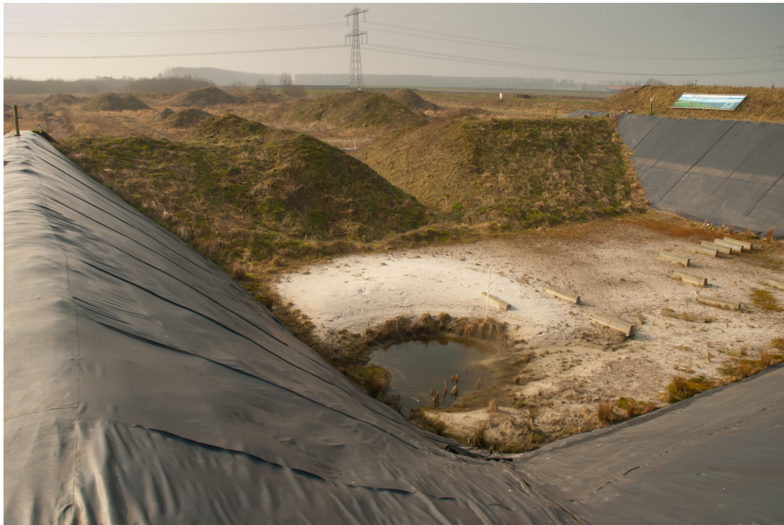
FIGURE A.5: Piping facility before reconstruction works
