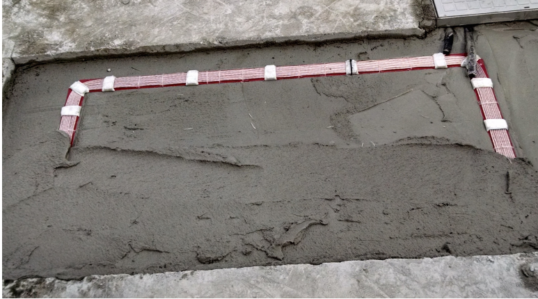
Figure 5.11: Road-embedding of the 9-turns WPT in dry concrete.
