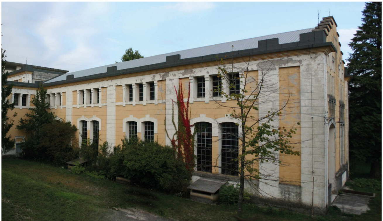
Fig. 4. Giais power plant. Left from the bottom: power plant plan, longitudinal section, western elevation windows detail. Right: architectural layout of western windows © F. Chinellato, L. Petriccione.
