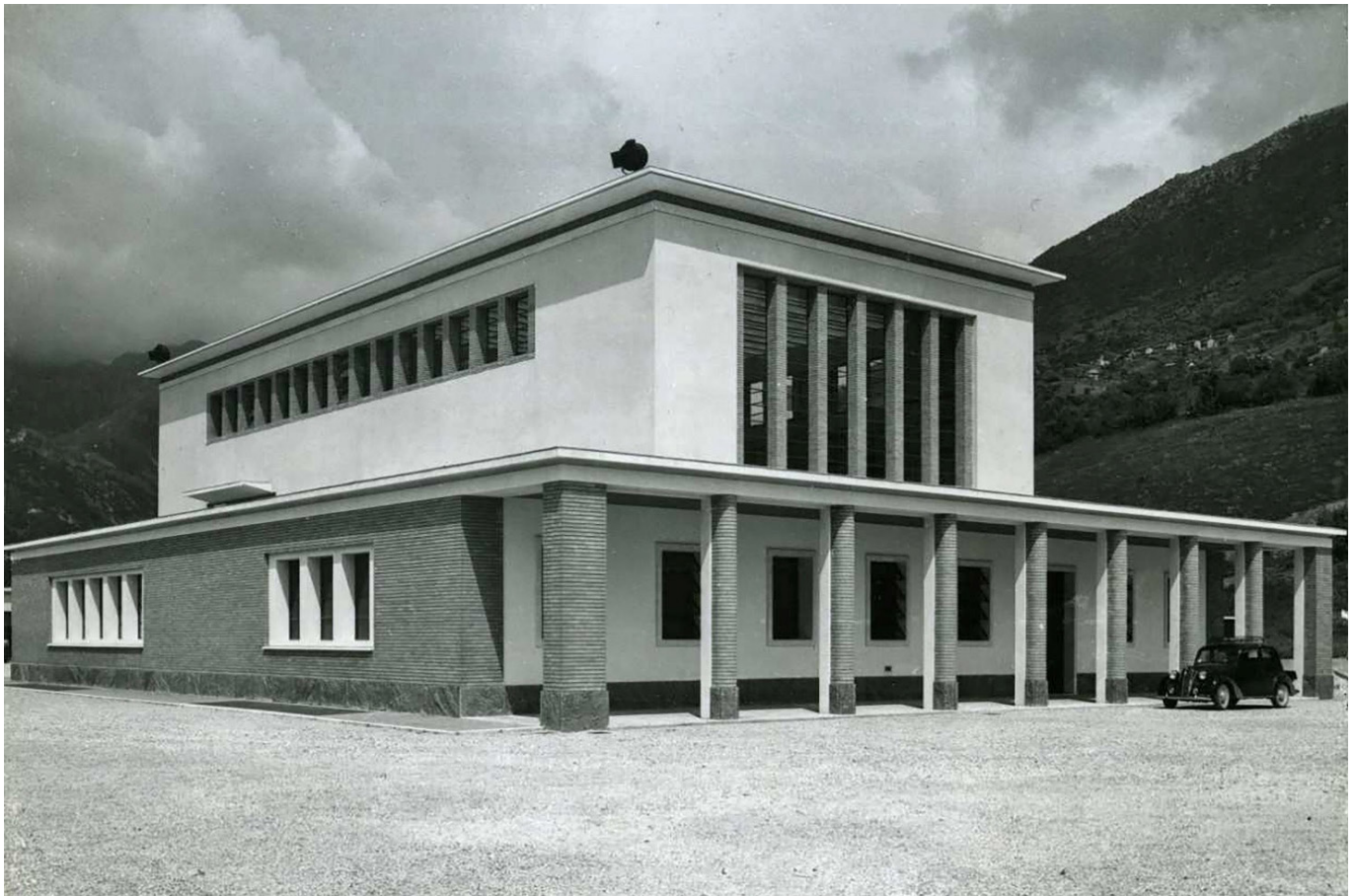
Fig. 9. Historical photo of Meduno power plant.
