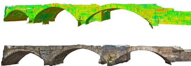
Figure 2. The point clouds of the bridge generated by laser scanning (above) and by SfM (below).
