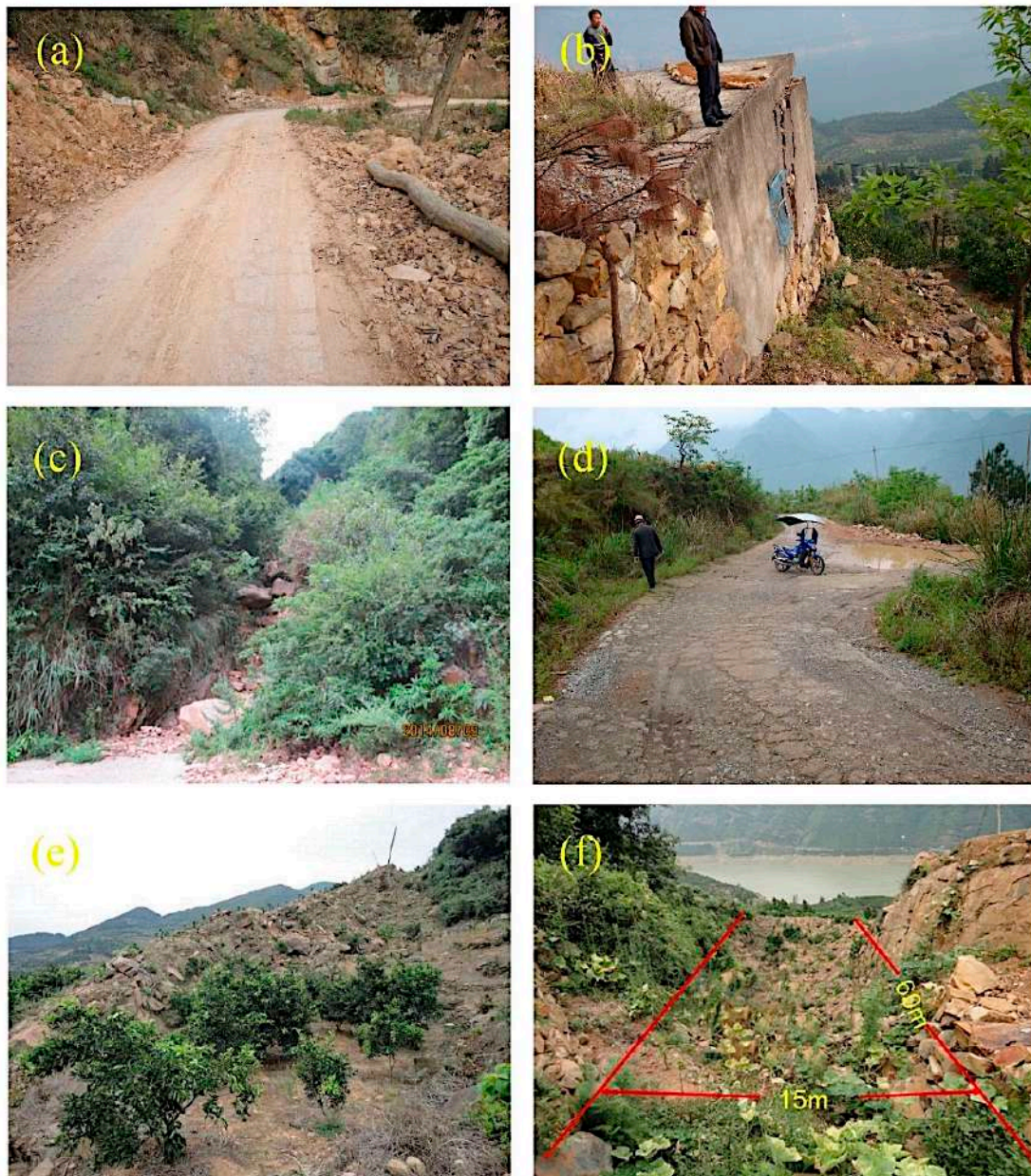
Figure 4. Deformations on the Muyubao landslide: (a) road damage on the west boundary, (b) deformation of buildings, (c) a local collapse on the west side, (d) road damage on the east side, (e) a collapse in the middle of the west side and (f) a tensile trench on the east side.
