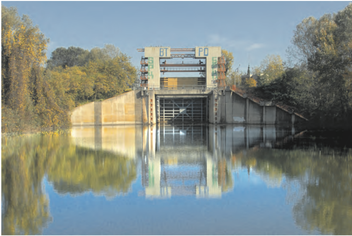
Fig. 4 - The sluice in Vigonovo (PD). (photos by S. Antoniadis, 2016).
