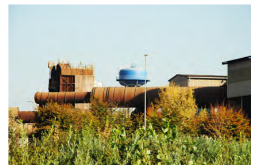
Fig. 3 - Industrial buildings and machinery aside the Padua-Venice waterway, steel factory (Acciaierie Venete). (photo by L. Siviero, 2016).
