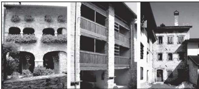
Figures 1, 2, 3 - From the left: the porch and loggia type, typical of the upper Valcellina, but generally present in the Carnic Prealps and in Carnia, the “balcony on pillars” type in a building in the Val Colvera and the “closed type” present above all in Cimolais and Barcis (Chinellato et al., 2002).
