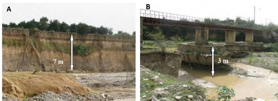
Figure 7. Channel incision due to in-stream gravel and sand mining (A); Effects of channel incision along the Talar River and effects on bridge stability (B) [57].
