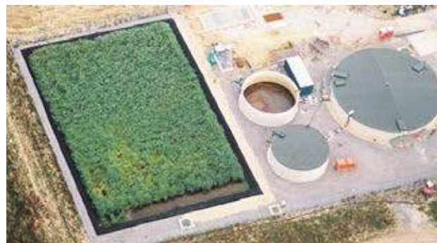
PLATE 2: General arrangement of the Leachate Treatment Plant and reed bed at Efford. (Robinson, 2018).
