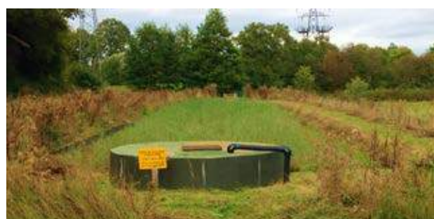
PLATE 1: General view of Shirley Reedbed from the inlet end, showing the Leachate Header Tank in the foreground, September 2014. (Robinson, 2017a).
