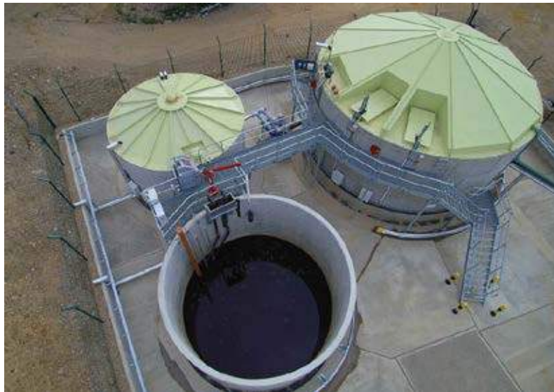
PLATE 2: Hatfield Leachate Plant: Detail of small roofed Raw Leachate Storage Tank, roofed SBR tank with twin venturi aerators on the right, and unroofed Treated Leachate Balance Tank.
