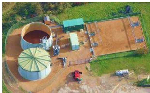
PLATE 3: Aerial view of the updated Small Dole Leachate Treatment Plant, following modifications made in 2010. (Robinson, 2017b).
