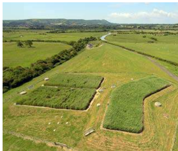
PLATE 4: Aerial view of the Small Dole vertical flow reed bed, and the two parallel horizontal flow reed beds, following construction by Phoenix Engineering in 2010. (Robinson T., 2017).
