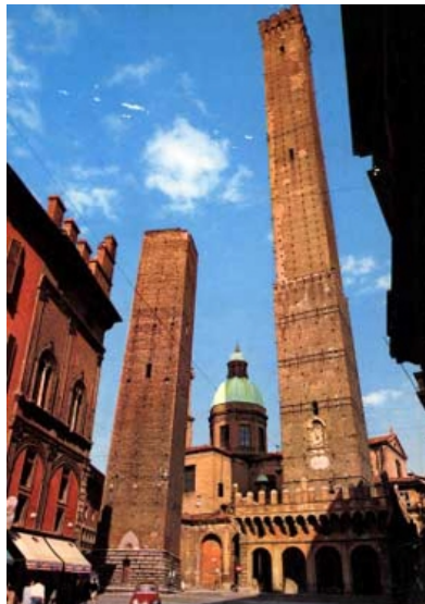
Figure 2 – Present picture of the “Two Towers” of Bologna. The Garisenda tower is the lowest one, on the left, while the tallest on the right is the Asinelli.
