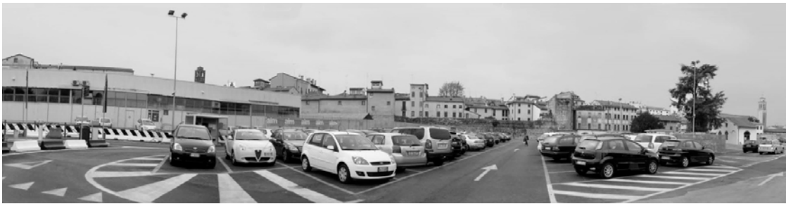
Fig. 3c. View of the case study area, current state (Pozzato 2012)
