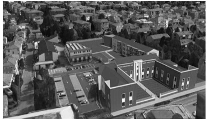
Figure 6 – Overview of the recovery project
