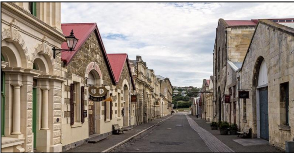
Figure 19: Harbour Street in Oamaru. The buildings were constructed between 1875 and 1885 using Oamaru limestone.
