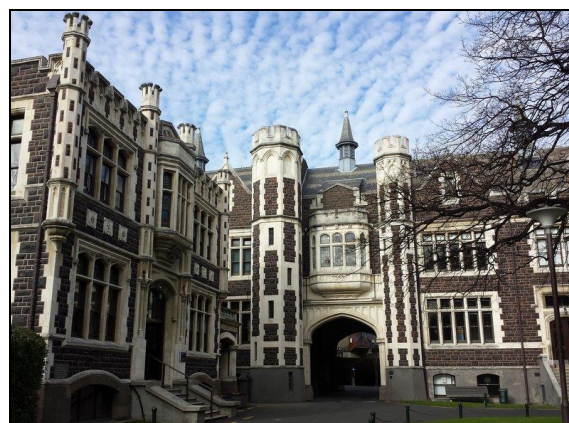
Figure 16: University of Otago in Dunedin. Built between 1878 and 1923 with Leith Valley trachyandesite and Oamaru limestone as ornamentation.
