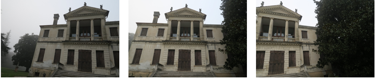
Figure 1: Panoramic-like image acquisition of the façade of Villa XXV Aprile, Mirano, Italy.
