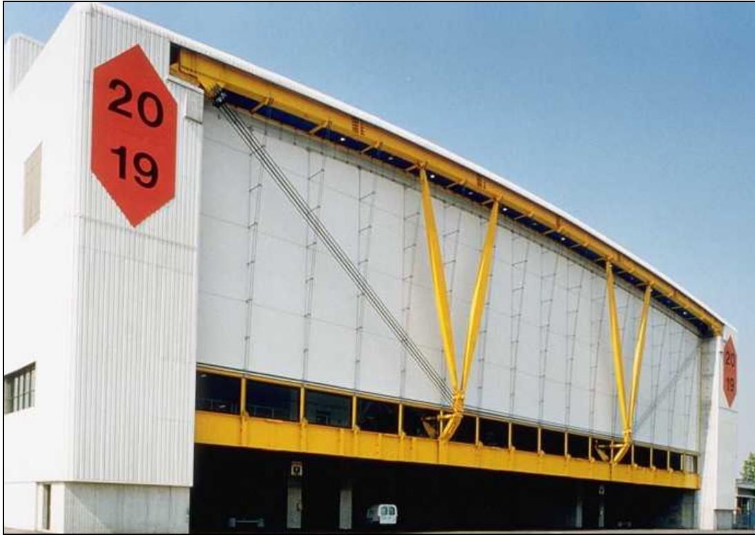
Figure 2: Pad 19-20: north façade.
