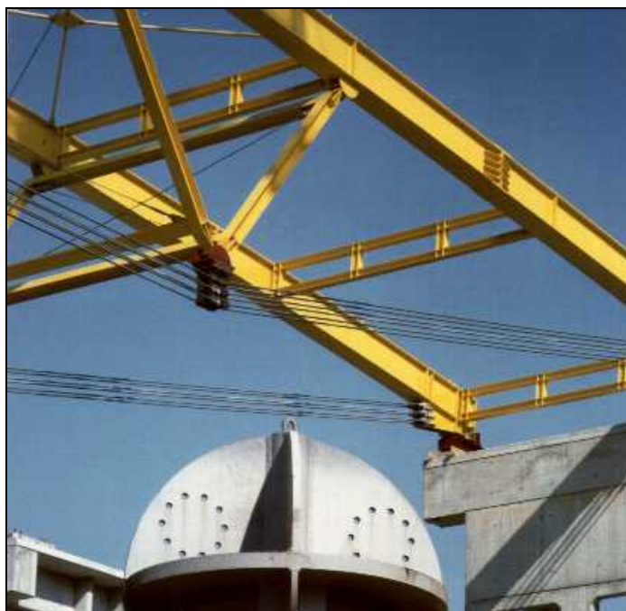
Figure 3: Upper arch-beams view.
