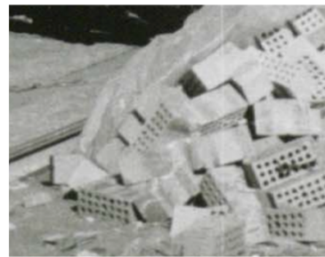
Figure 3: Hollow clay brick used for infill panels and photo of coeval school construction site.
