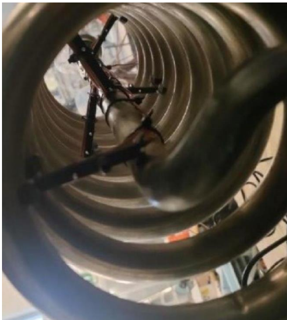
Figure 3. Sensors installed close to the coil
