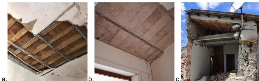
Fig. 5. Examples of diaphragms: a) flexible (timber joists); b) semirigid (steel joists and clay tiles); c) semirigid ceiling (r.c. joists and clay tiles) and rigid roof (cast-in-place r.c. ribbed slab).
