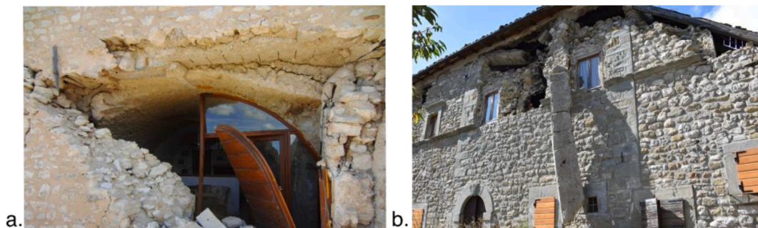
Fig. 1. R.c. ring beams added on historical masonry buildings: a) carved ring beam, at floor level; b) ring beam covering the whole wall thickness at roof level.
