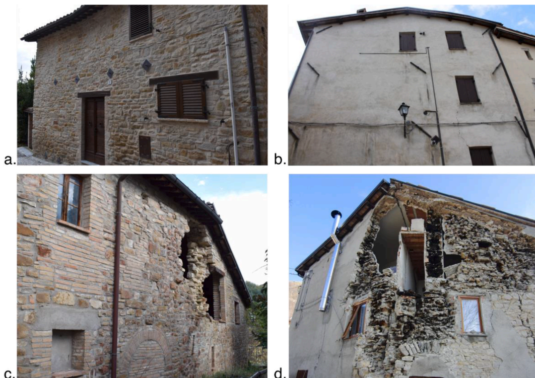
Fig. 3. Empirical effects of interventions on buildings: a) improvement ensured by joint repointing, strengthening of floors and tie rods; b) upgrading through masonry jacketing, tie rods and strengthening of floors; c) worsening owing to superficial repointing and replacement of floors with r.c. structures; d) downgrading caused by absence of interventions on walls and replacement of floors with r.c. slabs.
