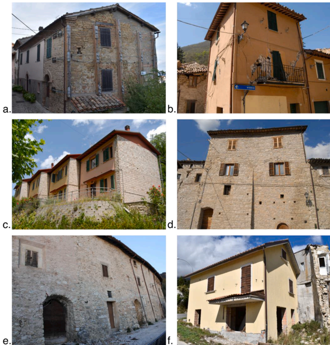
Fig. 6. Examples of building types: a) traditional (M1-F); b) hybrid with ineffective interventions (M1-S); c) modern (M1-R); hybrid with effective interventions: d) MIR-S, e) MIC-R; f) recent (M3-R).
