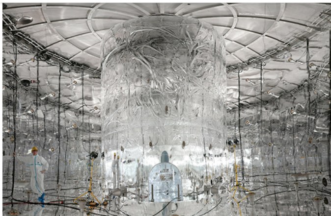
Figure 3.1: Inside the water tank after the installation of the muon veto system [46]. Photo from [47].
