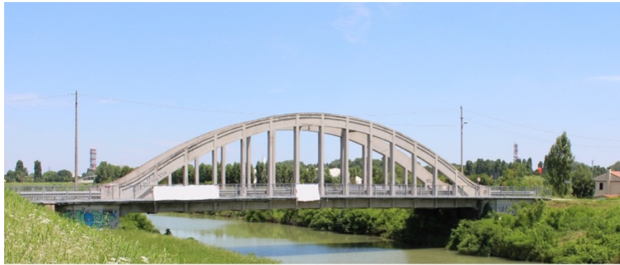
Figure 6: Case study – r.c. tied-arch bridge.
