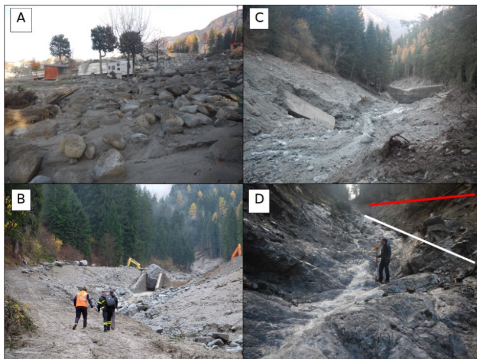
Figure 3.2: pictures of the post-event conditions. The debris deposit at the campsite (A), the sediment trap (B), the check dam channel reach (C) and the upper part of the channel (D); the white and red lines represent the minimum and maximum debris-flow front height with respect to the channel bed.
