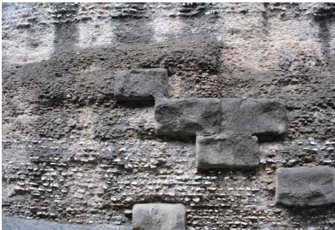
Fig. 5. Opus caementicium foundation of the Hadrian Mausoleum in Rome (today's Castel Sant'Angelo) in Rome (mid 2 nd century AD) (Dilaria in press).
