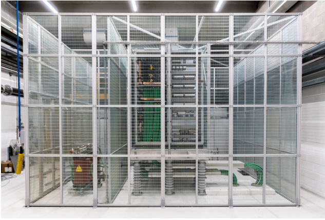
Fig. 3. The high-voltage platform designed to maintain the TIS unit at 40 kV in order to enable the isotope extraction.
