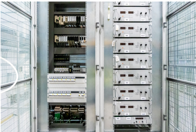
Fig. 4. The power supplies used to heat up the SPES target and ion source up to the nominal temperature of 2000 °C.
