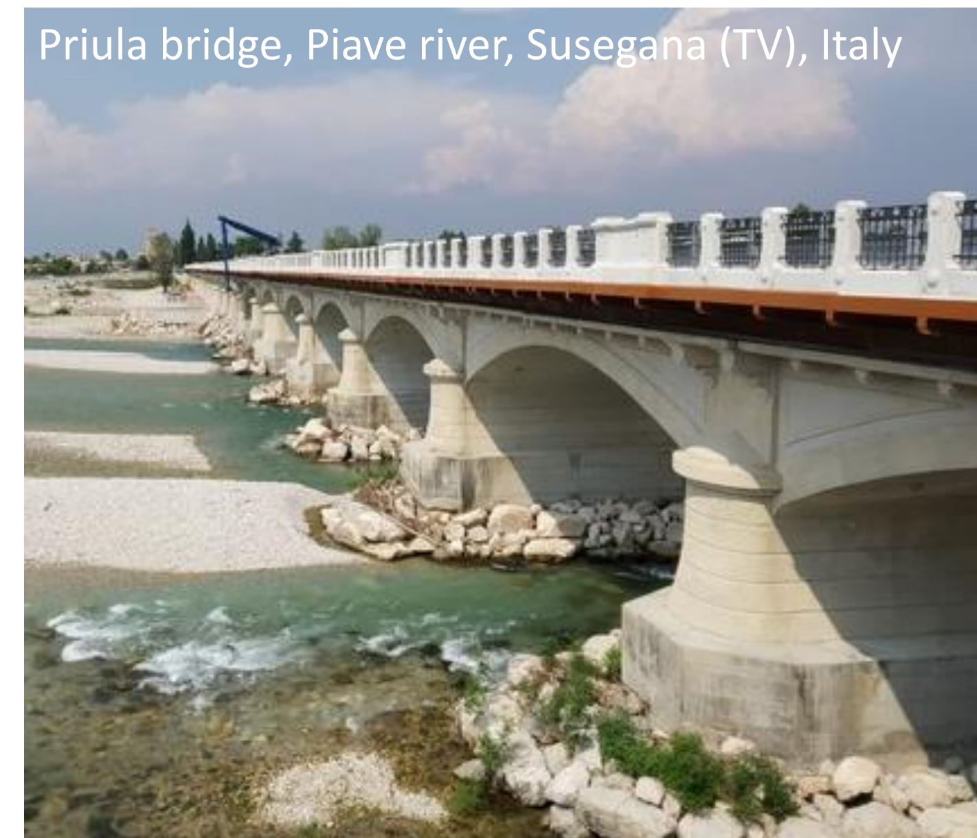
Priula bridge, Piave river, Susegana (TV), Italy Along the time, the rip-rap deepens in sand/silt riverbed material, assuming an inverted conical shape.
