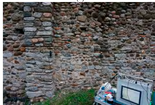
Figure 10. Setup of dynamic identification tests: (a) elevation of the grid for sensor positioning on the north wall and the apse; (b) view of accelerometers and acquisition system.
