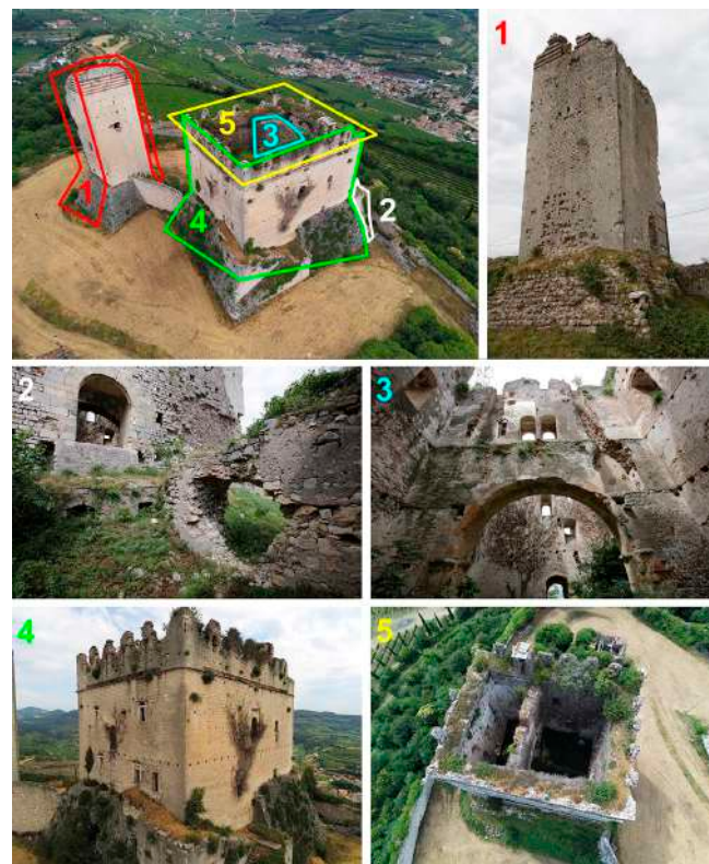
Figure 3. Characteristics of the tower and palace of Illasi Castle highlighting the complexity of the structures and showing the unremoved vegetation (1–5 show the portions enclosed by the colored polylines).
