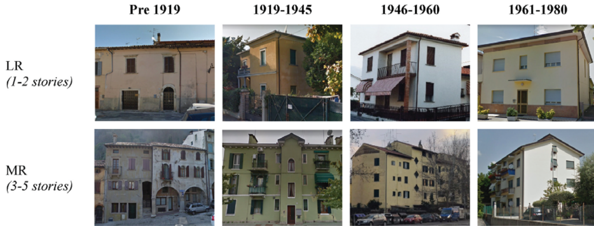
Fig. 1. Examples of Italian masonry buildings by construction period and height class.
