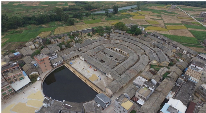
(b) Aerial view of the Hexinwu Building Complex
