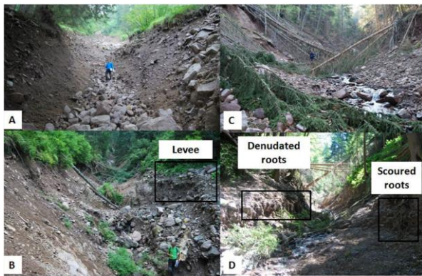
Fig. 2. Photos of the debris-flow torrents in the upper reaches (A), middle reaches (B), and lower reaches (C and D); field traces are highlighted in B and D.
