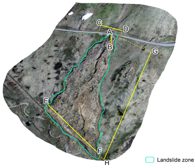
Figure 4.4. Details of landslide's features manually measured during the post-event field survey conducted in 2020. The 3D mesh was obtained through the UAV-derived point cloud data elaboration.
