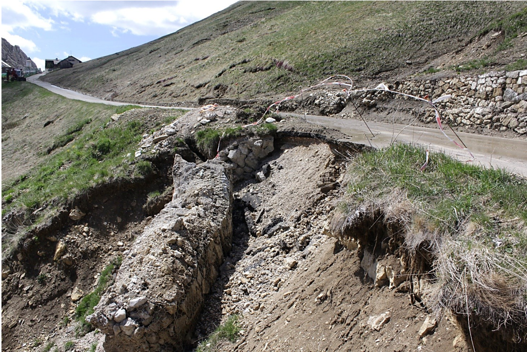
Figure 1.2 Example of shallow landslide activated above a section of a paved road located in a mountain grassland environment (Trentino Alto-Adige region, northern Italy; photo by Luca Mauri)
