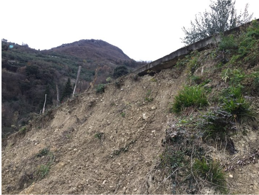
Figure 1.1 Landslide involving a slope under a section of a paved road located in a terraced vineyard in Trentino Alto-Adige region, northern Italy (photo by Luca Mauri)
