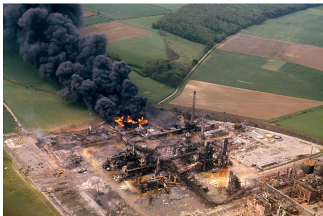
FIGURE 2 Nypro UK Flixborough chemical site after a cyclohexanone vapour cloud detonated (1974). PA/Alamy stock photo https://www.alamy.com/stock-photo-disaster-flixborough-explosion-nypro-uk-chemical-plant-north-lincolnshire-107574100.html
