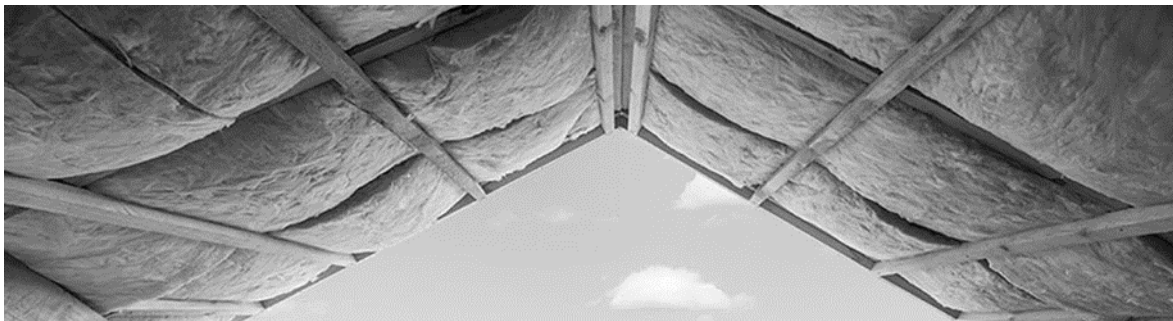
Figure 5. Example of sheep wool insulations on roof [41].
