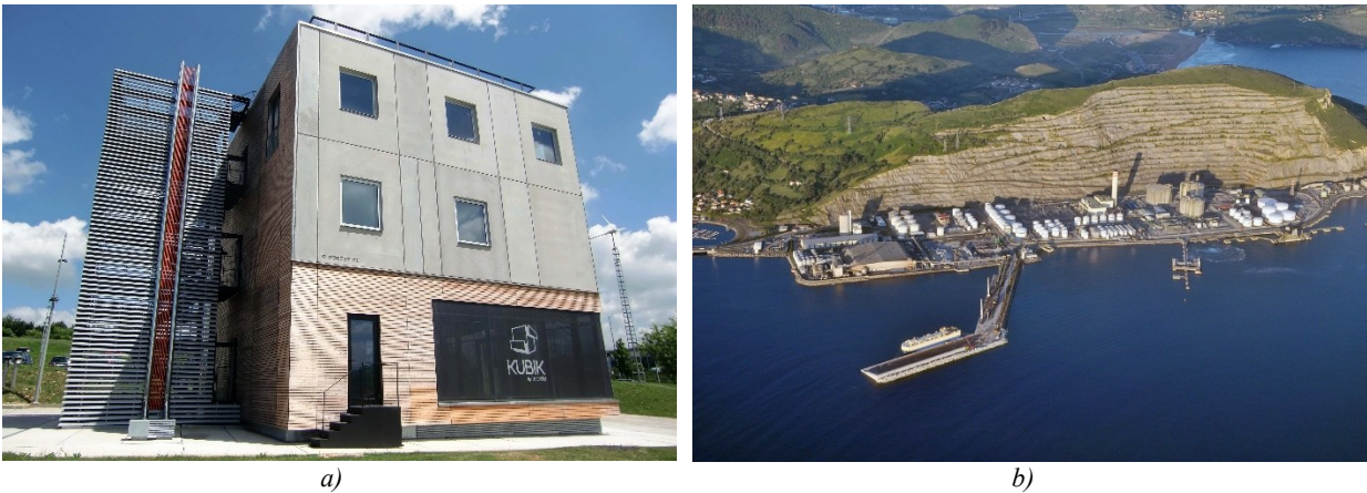
Figure 1-6. Applications of Electric Arc Furnace Concrete: a) KUBIK research building (Source: [102]); b) Port of Bilbao, Spain (Source: [101]).
