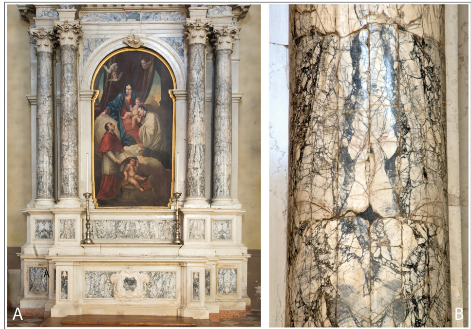
Fig. 5 A Madonna del Carmine altar in the Valli del Pasubio church. B Close view of a column. The mixture of marble and dark lamprophyre rock is prominent. The breccia was quarried in the eighteenth century in the Ronchetta Quarry (Mount Novegno), the same sampled by Giovanni Arduino
