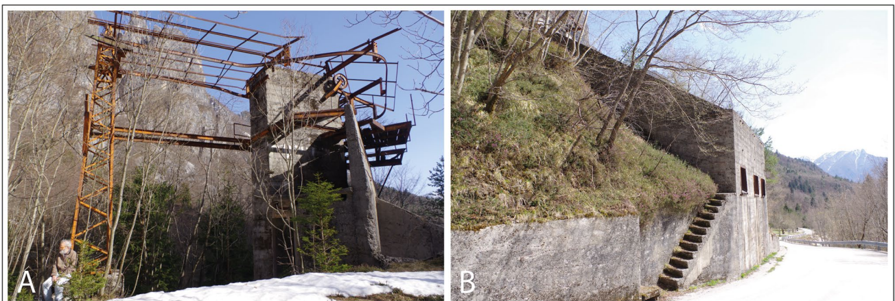
Fig. 8 A Arrival structure of the cableway, which before the asphaltting of the road served to lower the marble downstream. B The marble chunks were stored in the hopper, from which they were loaded onto trucks
