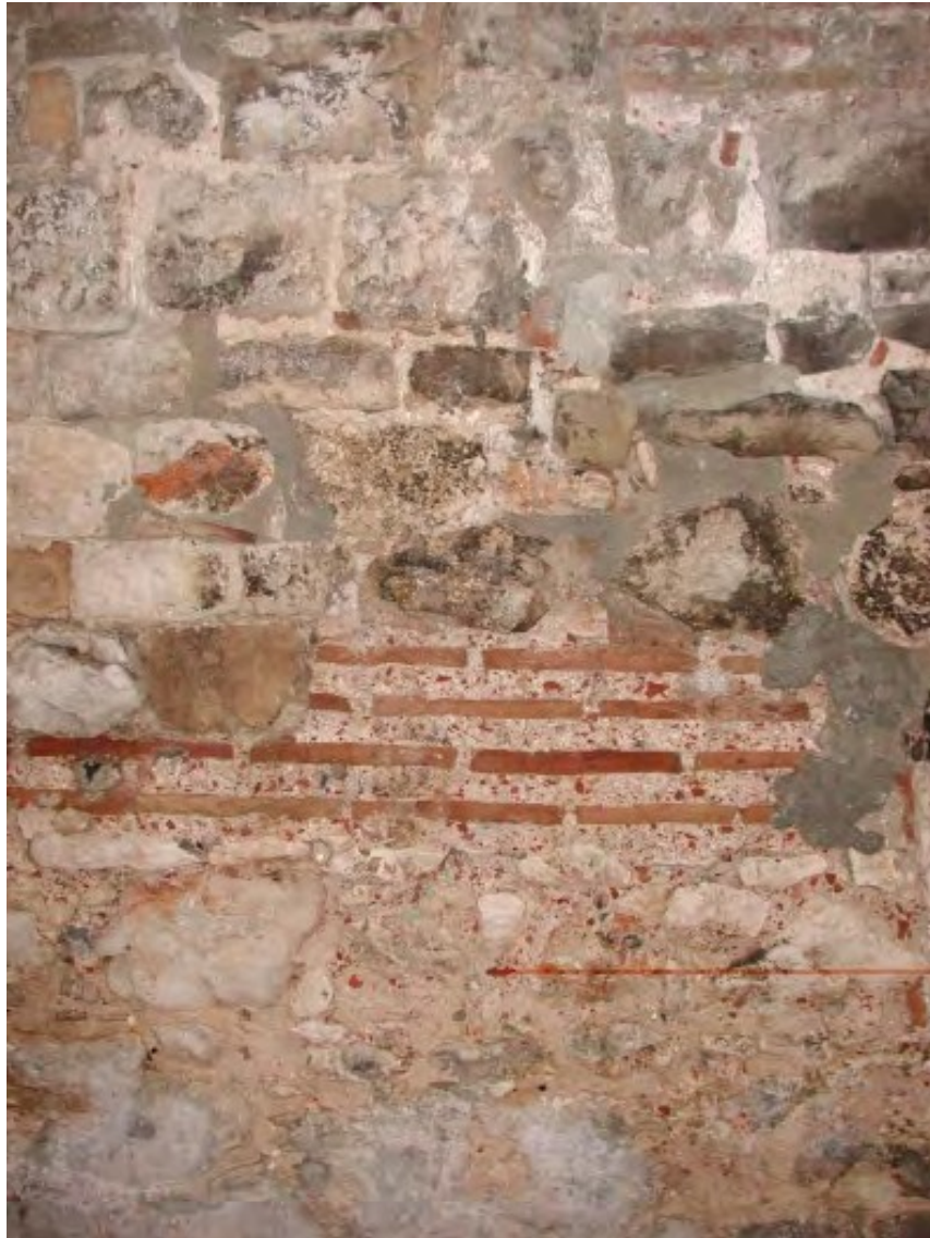
Fig.8 - Wall with inserts of Diocletian's masonry
