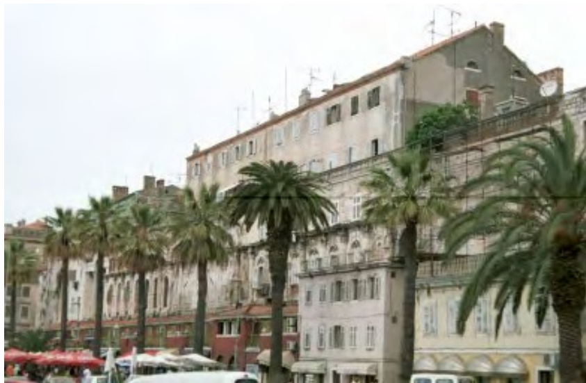
Fig. 2 - View of a part of the south-west wall of Diocletian's Palace
