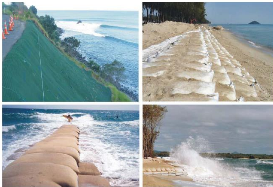
Fig. 3. Examples of geotextiles employment in civil engineering to protect the coasts (collection of free creative commons zero images).
