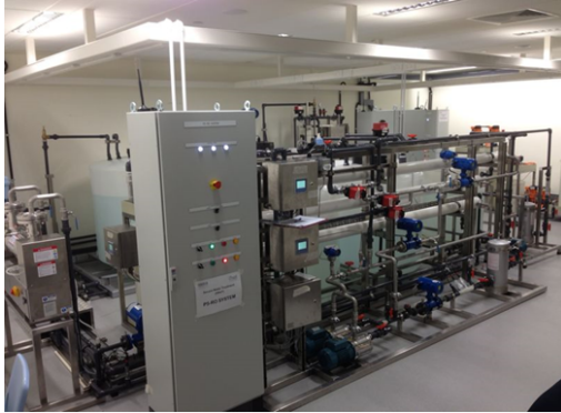
(a) SWaT Testbed by iTrust of Singapore.
