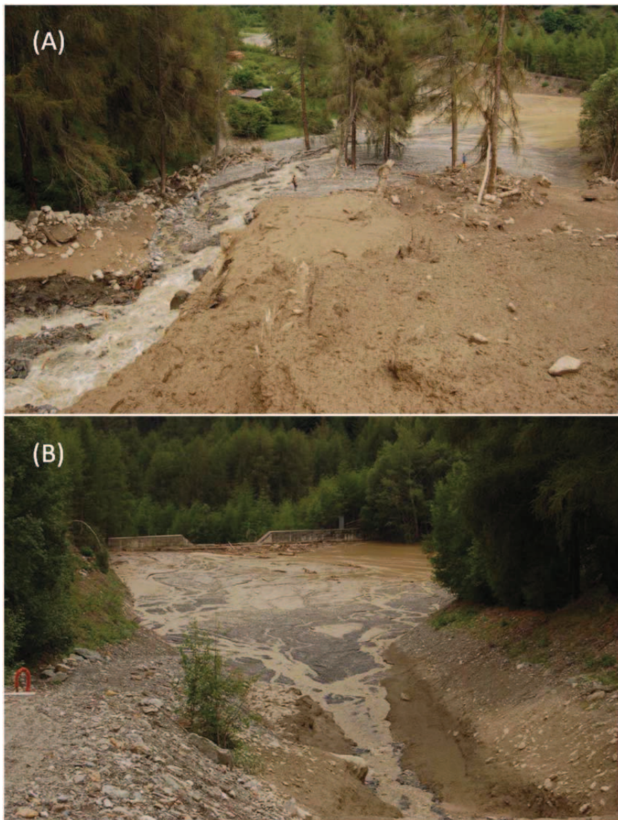
Figure 5. 13: Water and sediment input from Strimm river into the retention basin. upstream point of view of the water and sediment input of Gadria creek into the open check dam. Large woods comes from Strimm creek.
