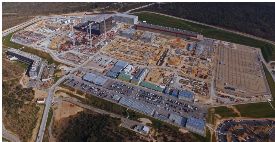
Figure 1-2 – Aerial view of ITER construction site, 2017
