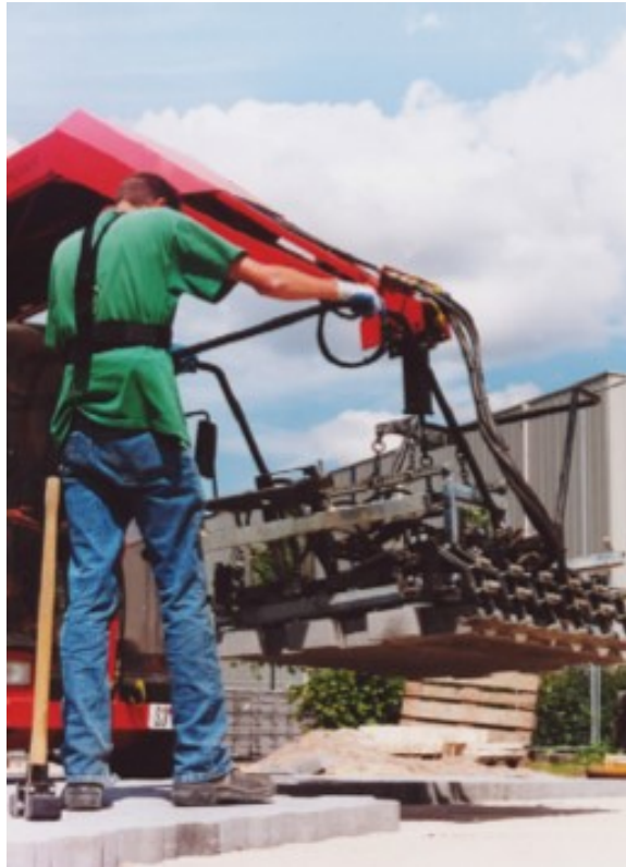
Figure 2.6 Machine with hydraulic clamp for brick assembly of floors (Burdorf et al. 2007).
