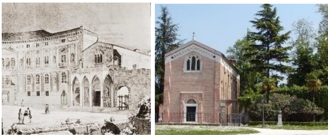
Figure 27. South-western façade of the Scrovegni Chapel. a) fragment of a historical engraving (1842) showing the facade with the portal in front of it [180]; b) current state of the façade [181]
