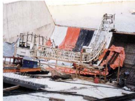
(b) St. Mary's Dam, Alberta
