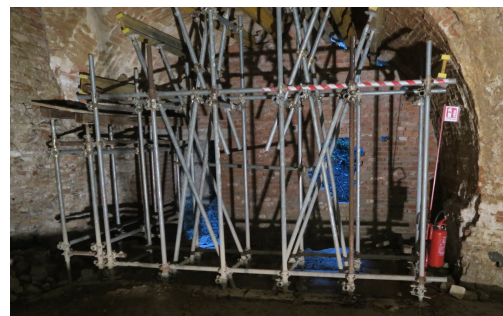
Figure 10. Final part of bastion left wing.
